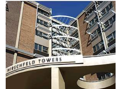
Hirschfeld Towers - Denver, CO
